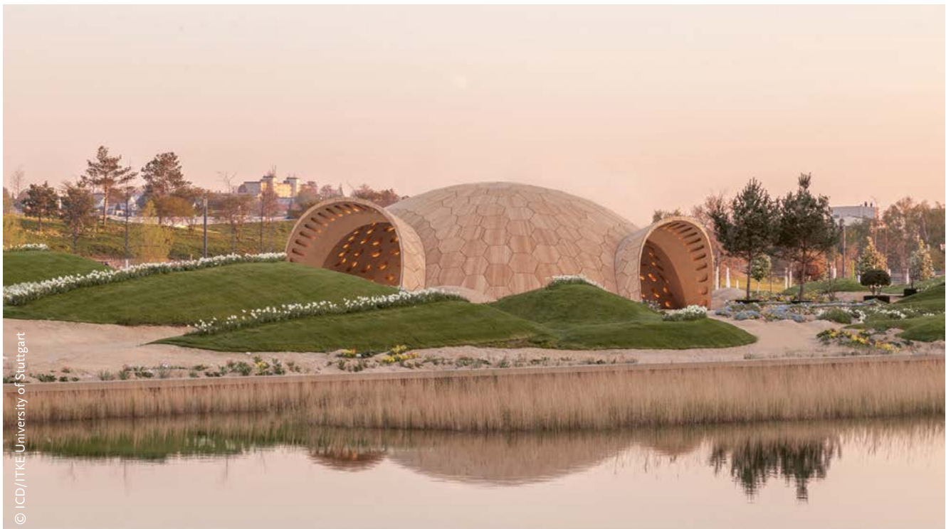
FIGURE 2: The dawn of a new material culture? BUGA Wood Pavilion at the National Horticultural Show 2019 in Heilbronn, Germany. The building was digitally designed and robotically prefabricated by the Institute for Computational Design and Construction (ICD) and the Institute for Building Structures and Structural Design (ITKE) at the University of Stuttgart: www.itke.uni-stuttgart.de/research/built-projects/buga-wood-pavilion-2019 .
